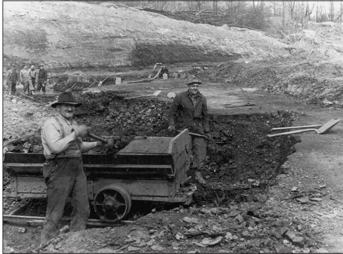
Early surface mining consisted of extracting coal that was exposed along a hillside, using picks and shovels (from Crowell, 1995, p. 18).
